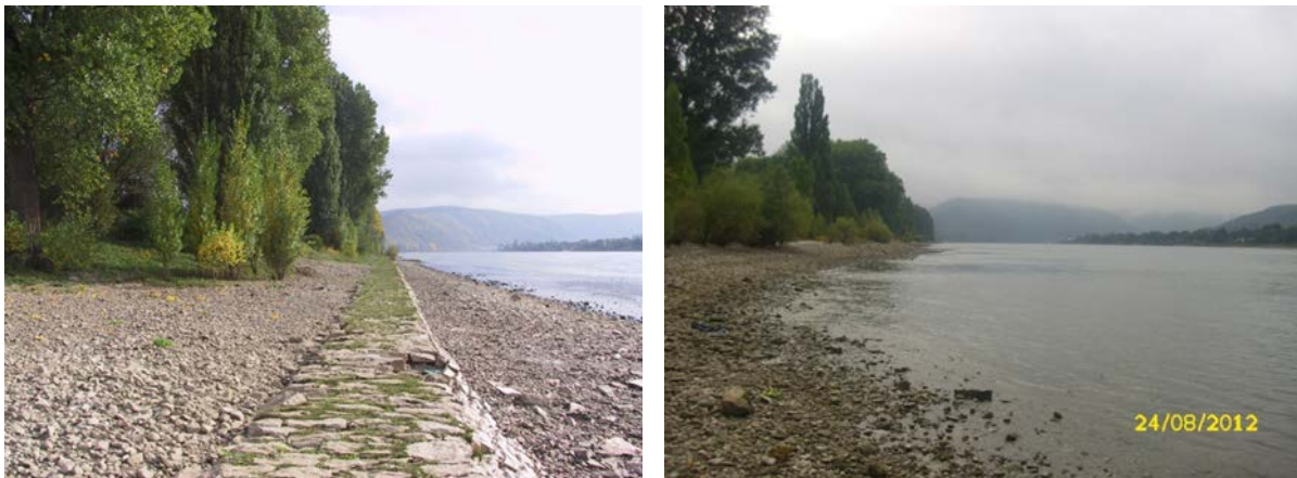
Figure 40: Bank of the Rhine before (left) and after (right) structural improvements - from reinforced banks towards flat river banks (photos: Angelika Halbig, BCE; Ernst-Dieter Kuczera, SGD Nord).
